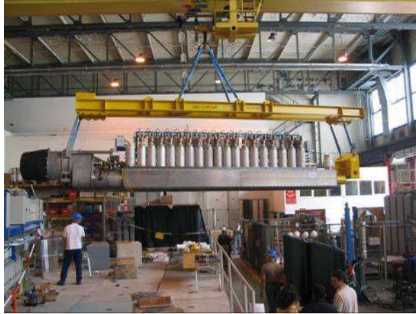
Figure 6: One of the biggest of the DFBs being lowered into the tunnel.
